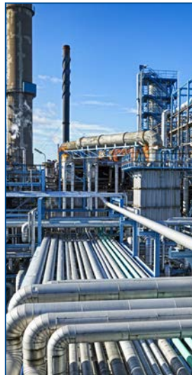
LONG PIPING RUNS WITH HIGH FRICTION LOSS
